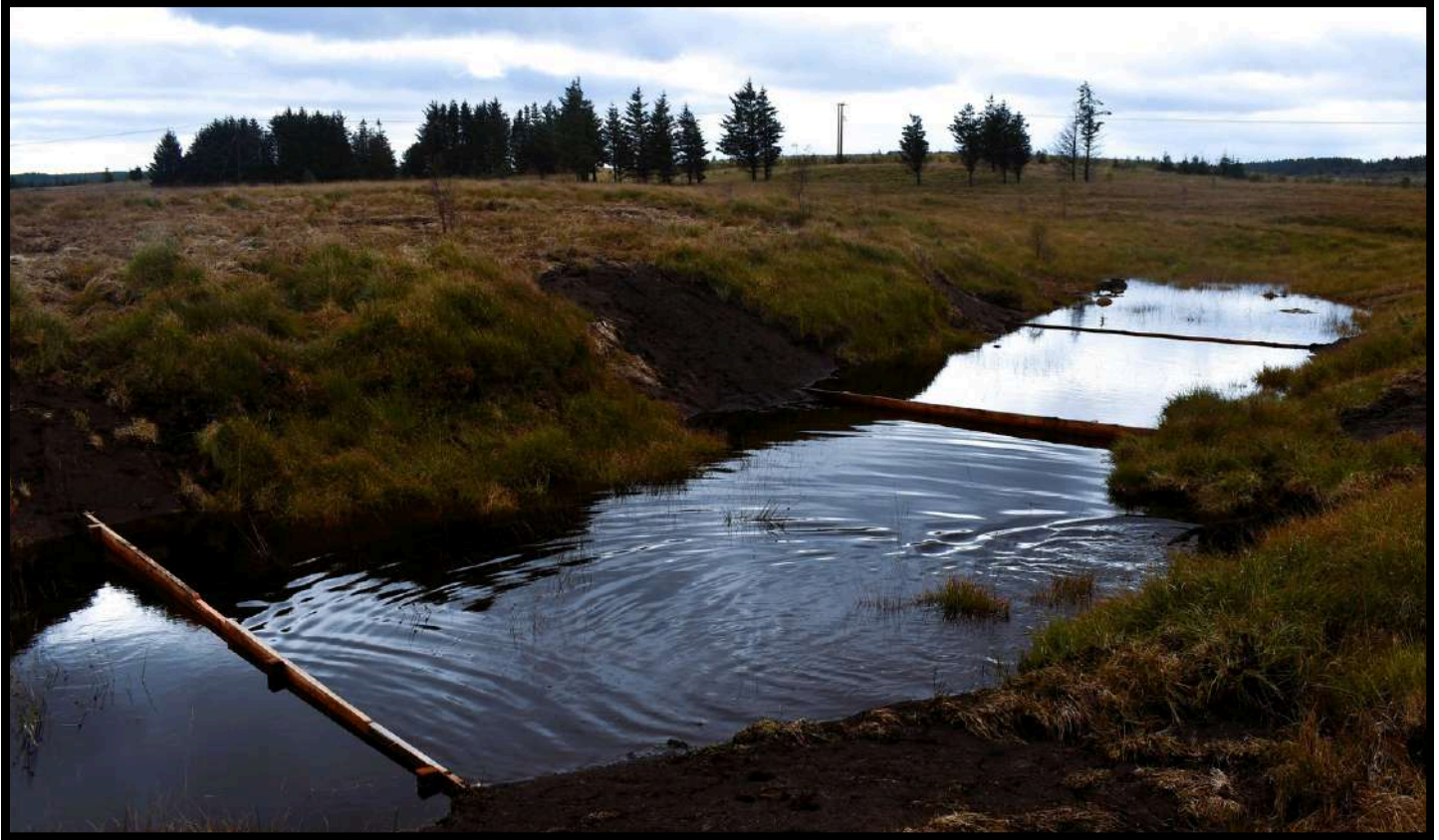
Timber dams: Blocking drainage channels and eroded areas
