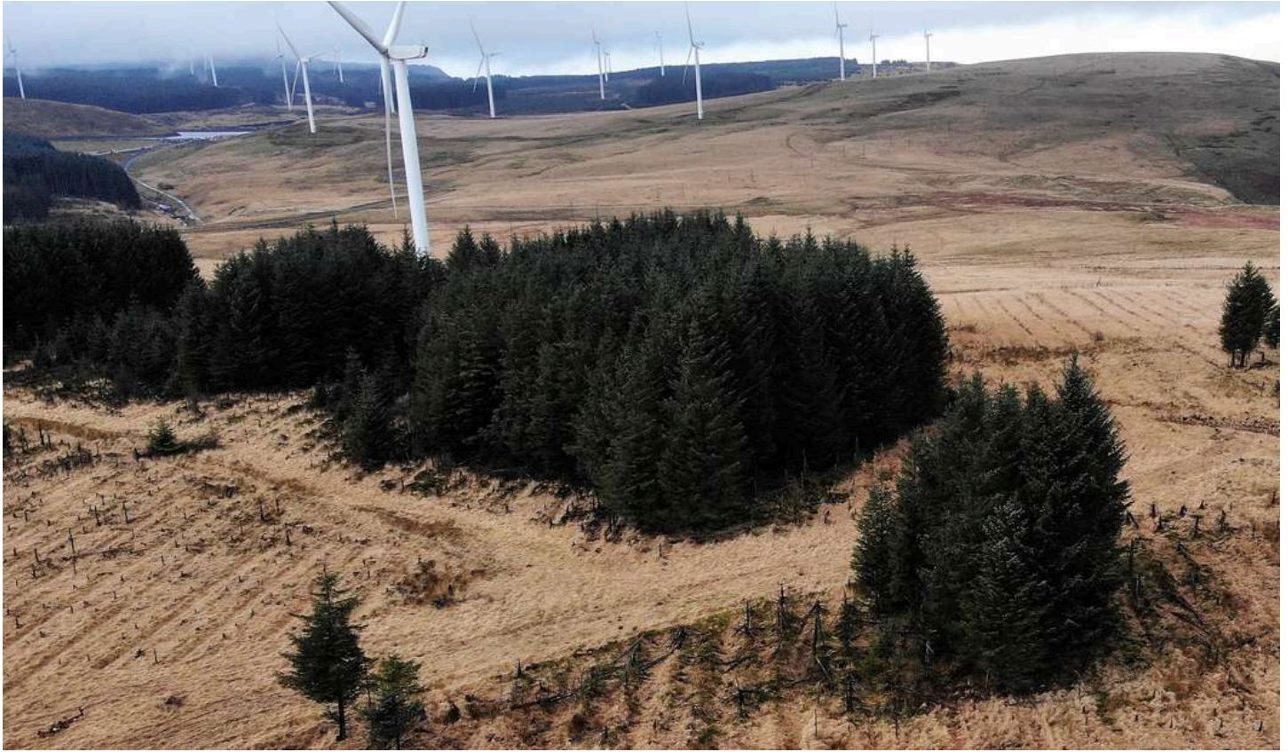
Castell Nos: Aerial View
